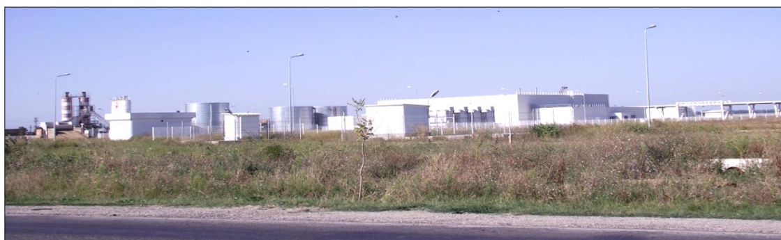
Figure 3. Wastewater treatment plant Titu - Sălcuța (Source: authors)
