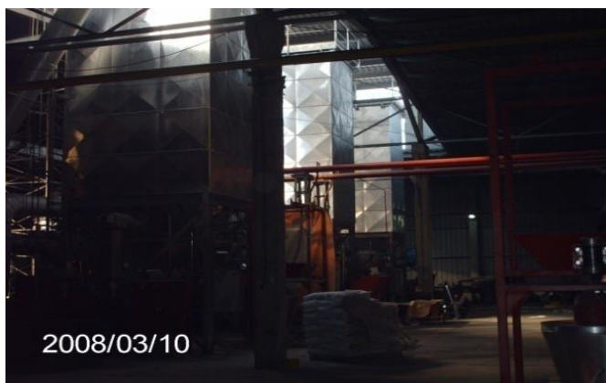
Figure 3 Cleaning System of the Burning Gases (Photo: Ana Humeniuc).
