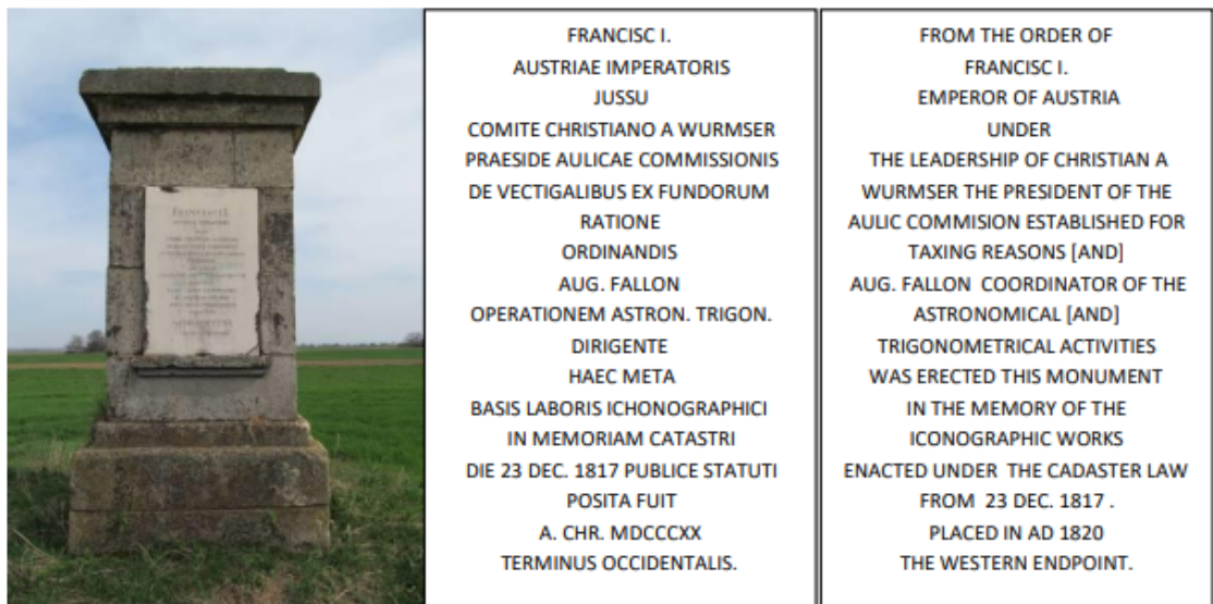
Figure 5 The monument erected in the western endpoint of the Rădăuți baseline (W.B.E.P): the reference point of cadastral coordinate system of Bukovina.
