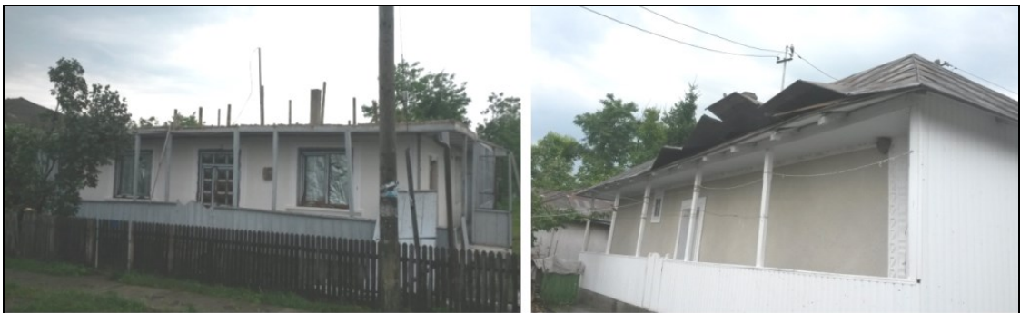
Figure 5 Building with roof separated and carried 150 m (left), and another building with a tin roof separated upwards (right).
