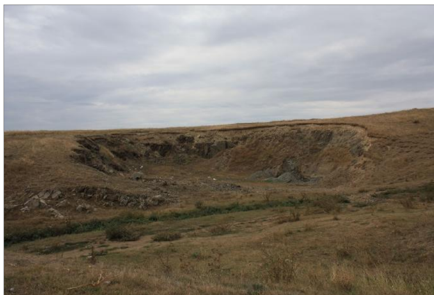
Figure 6. Compaction and pipping.
